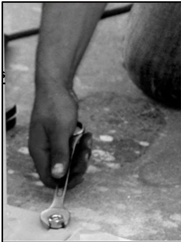
Figure 19 Secure Anchors with Wrench for Final Attachment
